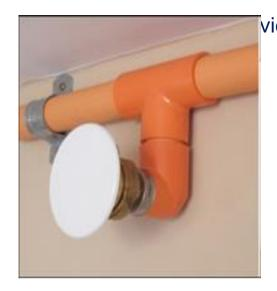
vided to confirm compliance. The 2 images are indicative of how the sprinkler would be installed within the corridors of each flat. The image to the right shows the concealment of the pipe work within a "Pendoc" trunking product.
