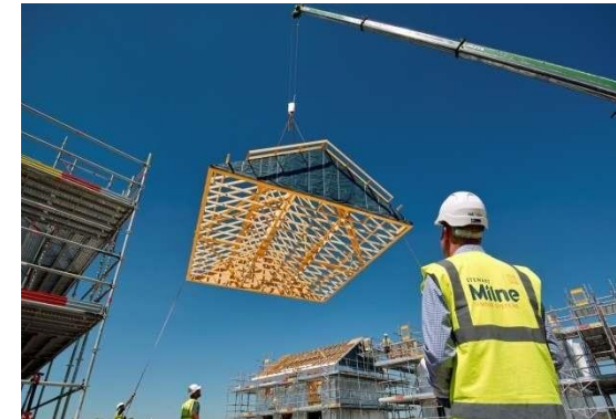
GROUND LEVEL ERECT ROOFS
