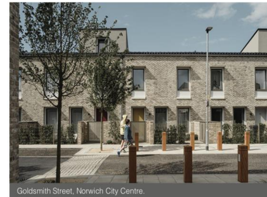
Goldsmith Street, Norwich City Centre.
